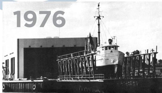
Link Engineering Laboratory building and Marine Shipping Railway built.
